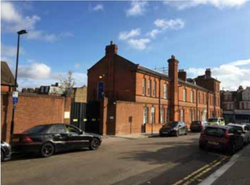
View east along Harold Road showing vehicle access
